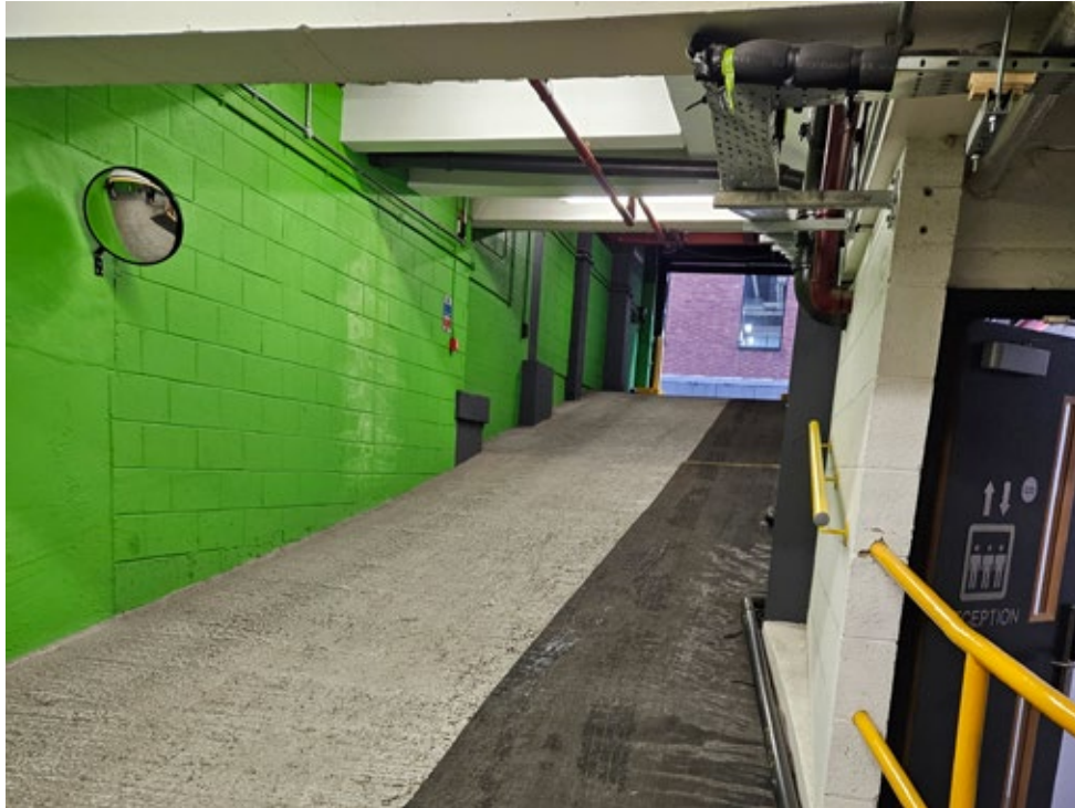
Ramp down to basement level
