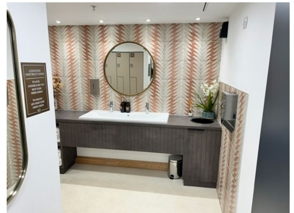
Vanity to changing area / shower finished to high quality and provision
