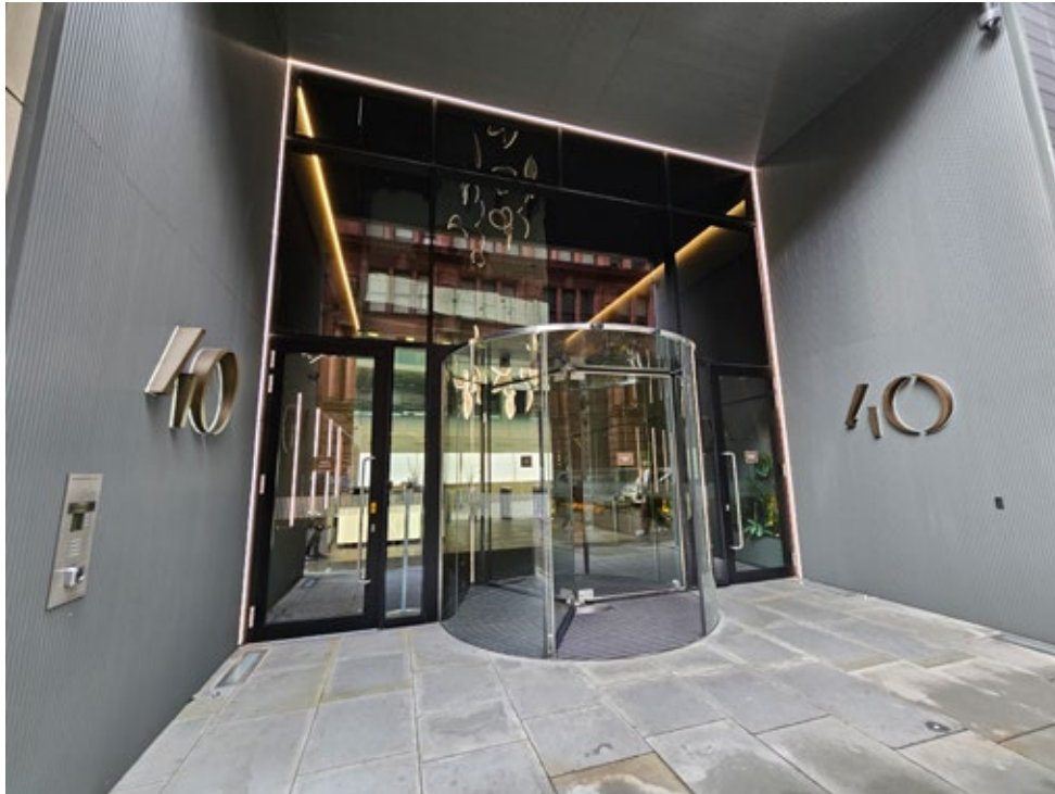
Main entrance revolving doors, similar to 55 Spring Gardens, but set back with large space in front for arrival and inviting users in
