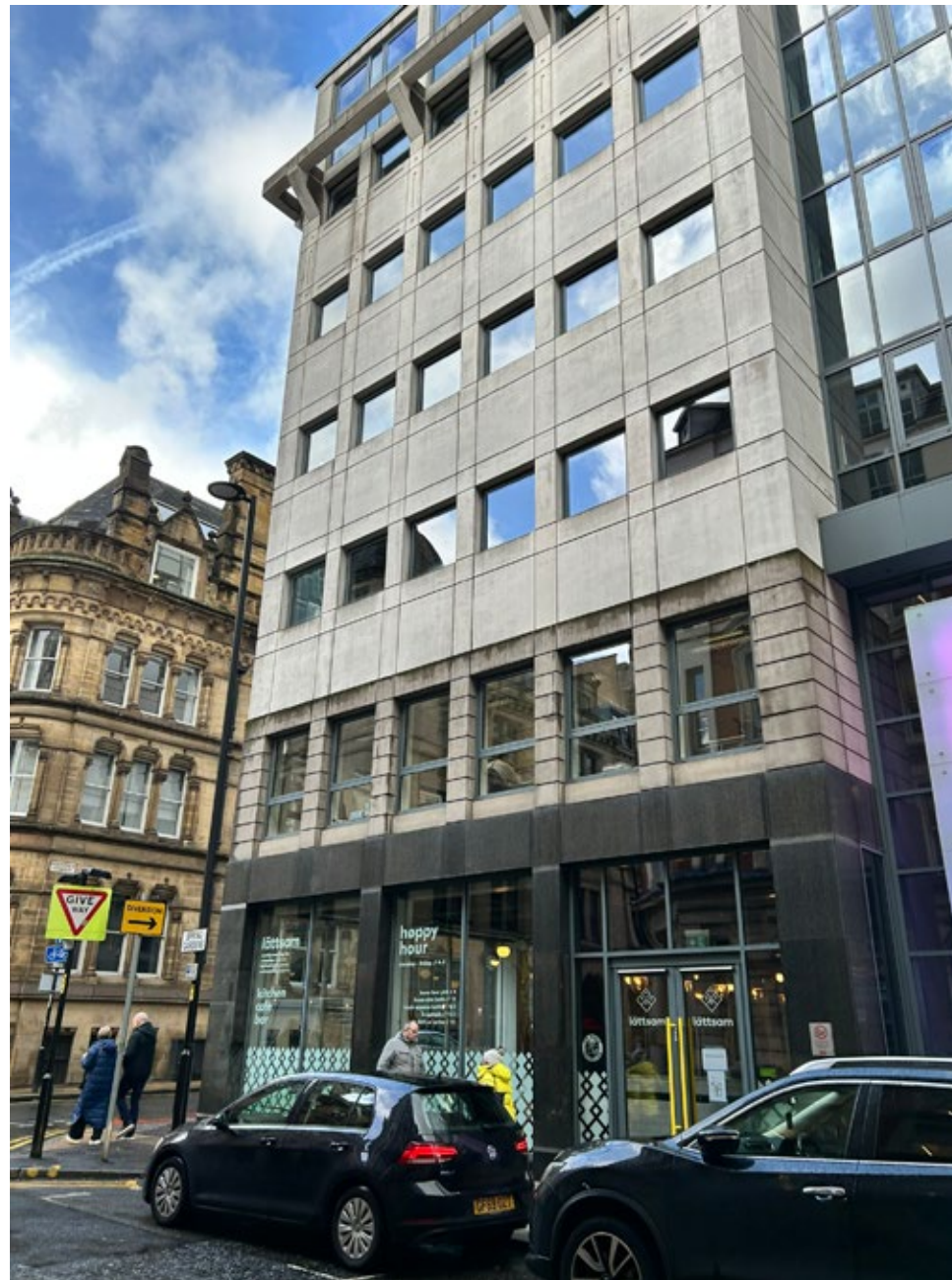
View from Spring Gardens / Fountain St corner
