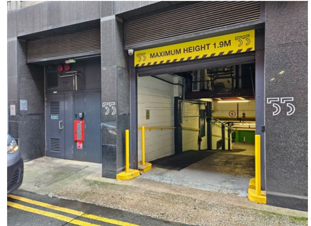
View of W. Mosley St basement car park entrance
