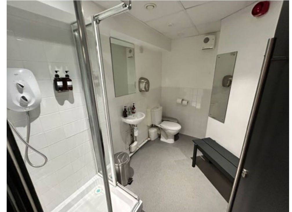
One of the basement showers for cyclists
